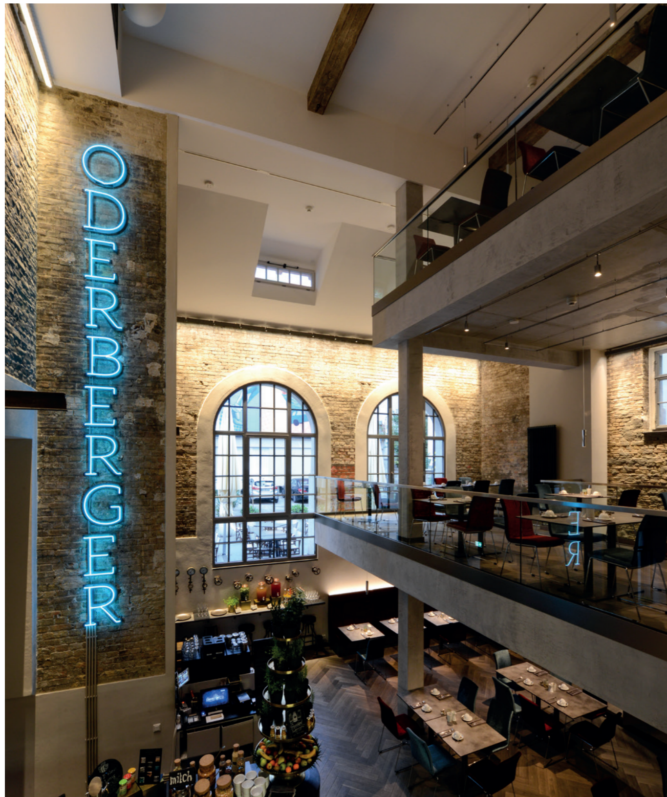
The historic Public Bathhouse "Volksbadeanstalt" in Oderberger (Germany) was subject of a total transformation and is now a modern swimming pool, with a spa and a 4-star hotel that includes a restaurant, a bar, several training rooms, 70 rooms, two apartments and five tower suites.
